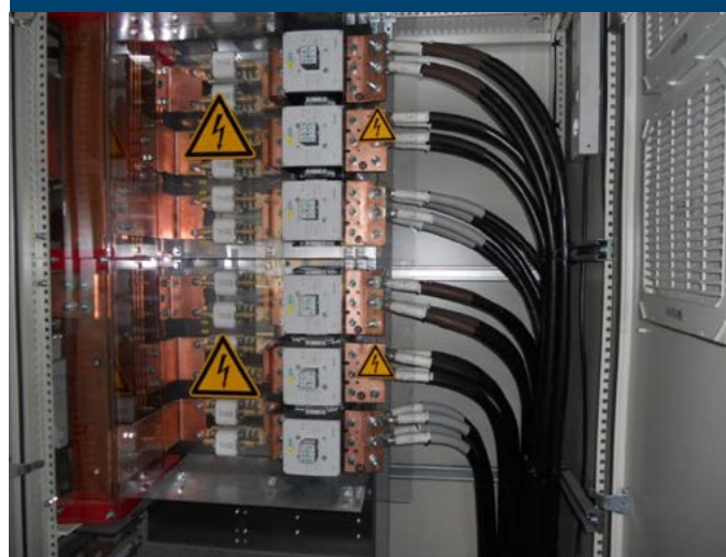
Fig. 8: Example of panel in machinery house with cable protection fuses
