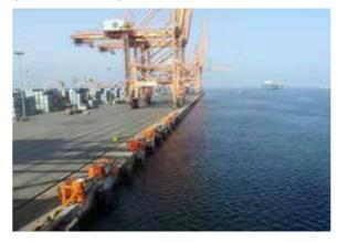
Port of Salalah in Oman experiences significant long wave impact during the monsoon season (Khareef season). To counteract these long wave effects, automated mooring systems were installed to dampen vessel movement while berthed. With the automated mooring system installed, it allowed the port operator to continue full loading/unloading operations even during the most severe long wave conditions while maintaining high efficiency.
