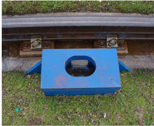
Photograph E: RMG crane pin socket
