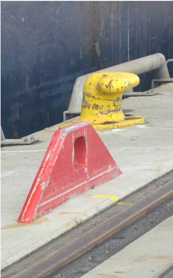
Photograph D: Combined tie-down and stowage pin socket
