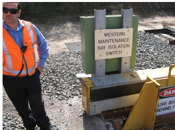
Photograph V: Power disconnect location for RMG crane powered by protected ground level bus bar
