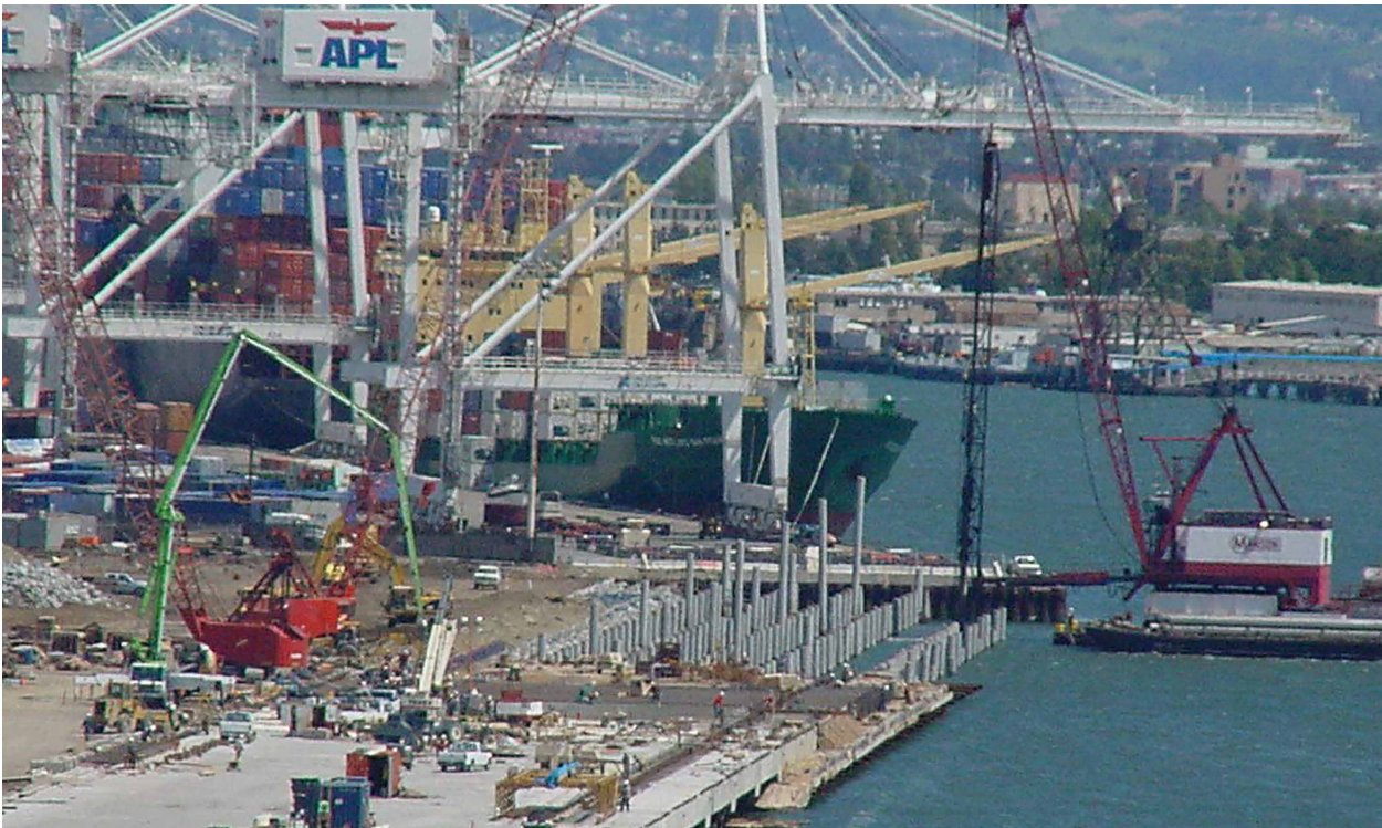
Photograph C: Construction of STS container crane wharf
