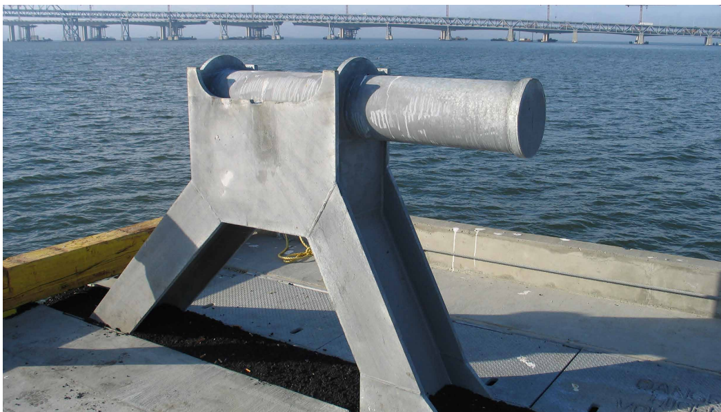
Photograph N: STS crane end stop without buffer
