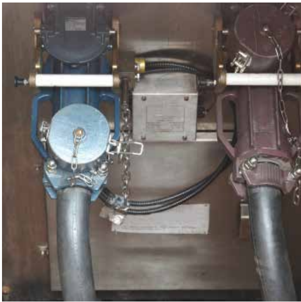
Picture 1: Example 6.6kV plugs for container ships and tanker vessels
