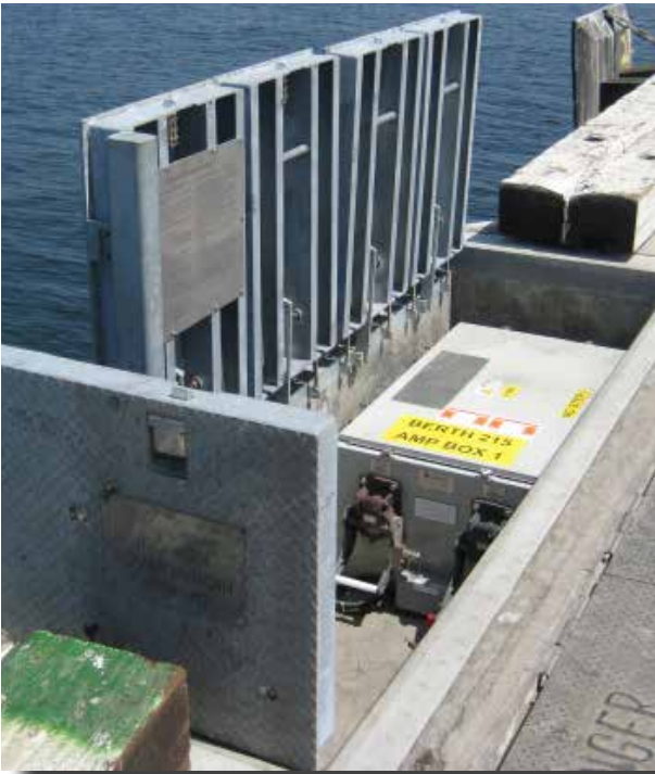
Picture 12: Fixed socket: in-ground socket outlet Junction Box with easy lift covers
