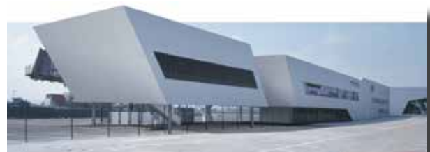
Picture 5: 12MVA Substation for cruise vessels at the Port of Hamburg. (Input: 10kV-50Hz, output: 6.6kV/11kv-60Hz).
