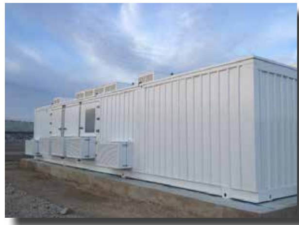
Picture 4: A 2MVA substation for a container vessel with static frequency conversion.
