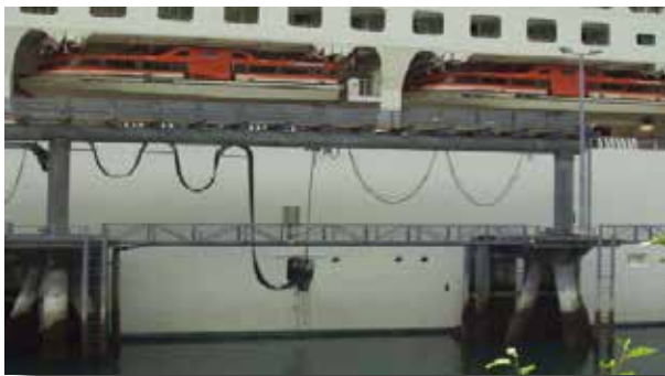
Picture 9: A festoon system mounted on a stilt structure
