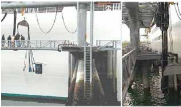
Picture 16: An alternative CMS for cruise ships incorporating a large saddle for cables that are hooked on a small crane. The plugs are caught from the vessel and pulled inside for connection
