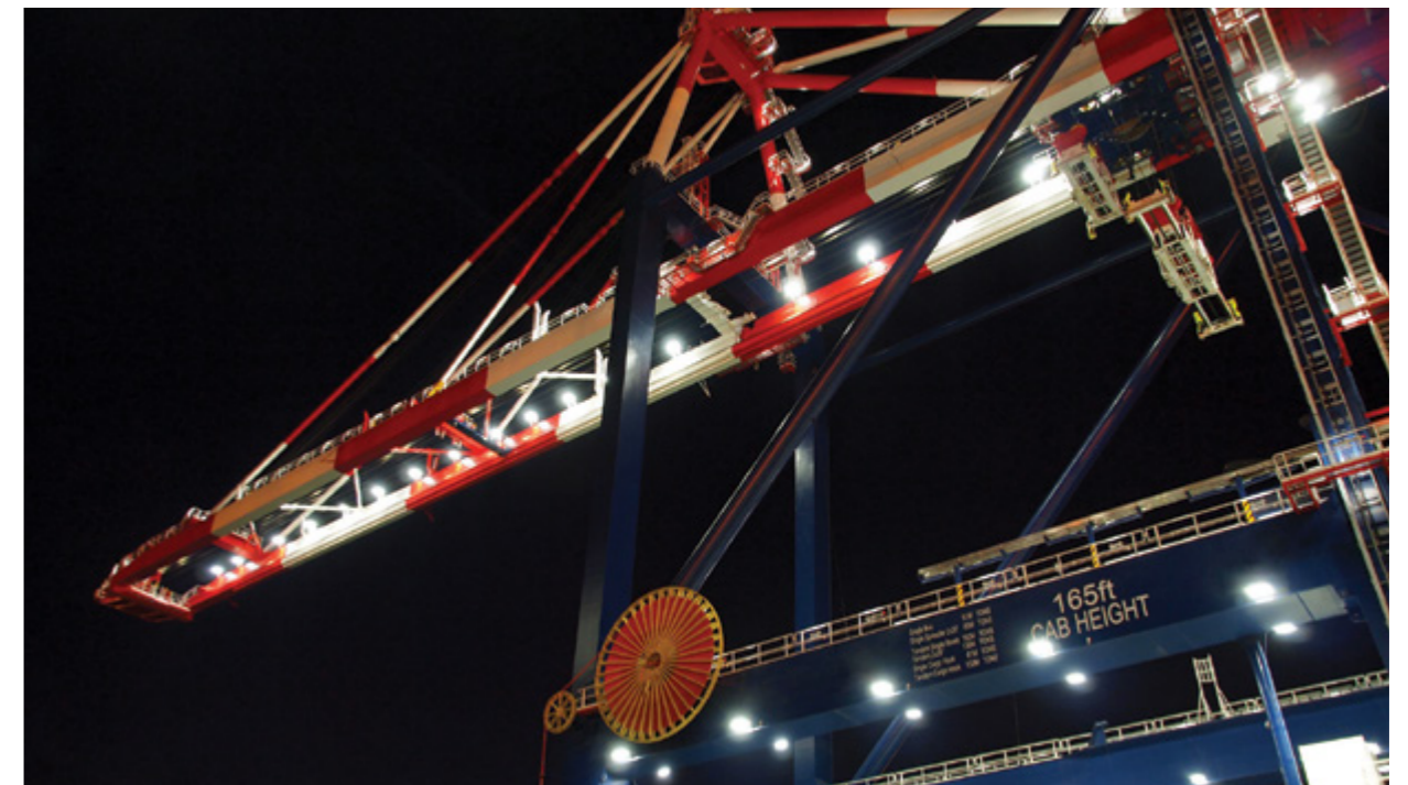
LED Floodlight illuminating STS crane at Long Beach Container Terminal in Los Angeles, CA
