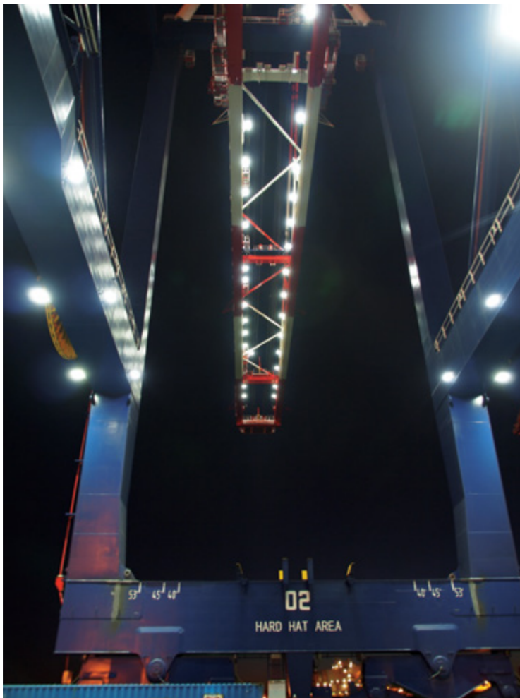
LED Floodlight illuminating STS crane at Long Beach Container Terminal in Los Angeles, CA
