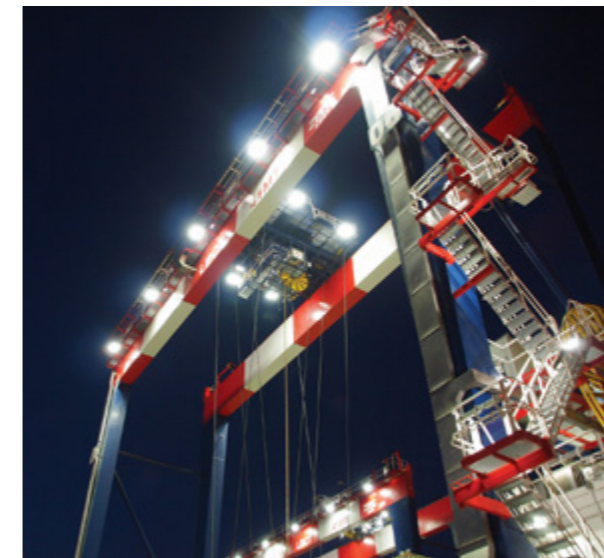
LED floodlights illuminate an ARMG crane at a US port
