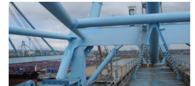
Picture 3.22: LS TGSB of a truss boom crane, in this case without radii at the points of transition.
