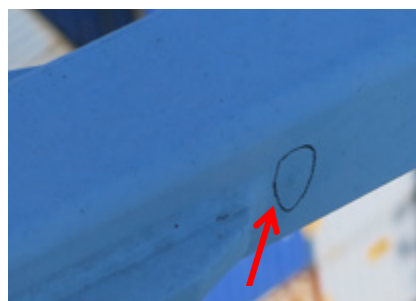
Picture 3.72: Washing and festoon platform hanger at end of girder. The arrow points to a crack indication at the end of the connection plate. The platform is lightly loaded, but bounces up and down during operation.
