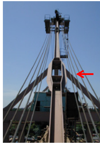
Picture 3.48: A geometrical discontinuity in the forestay. This area will have severe stress concentrations.
