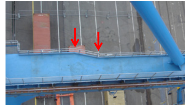
Picture 3.8: Portal beams with tapered end sections. The arrows indicate the transition points. The change in direction of the load in the web plates means there can be a significant cyclic tension load in the internal diaphragms.
