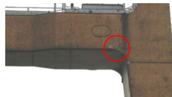
Picture 3.10: Another type of portal beam crack.
