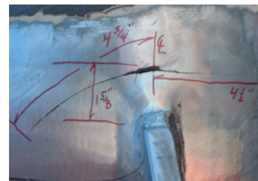
Picture 3.43: Dangerous cracks in an upper diagonal member. The member can fracture at any time.
